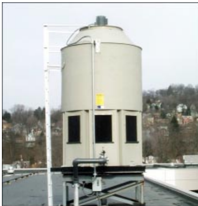
Built-in pockets reinforce the tower bottom so that the tower can be easily mounted on standard I-beams or imperfect pads. An engineered-plastic cooling tower used at the Conair plastics processing plant in Pittsburg, Pennsylvania.
