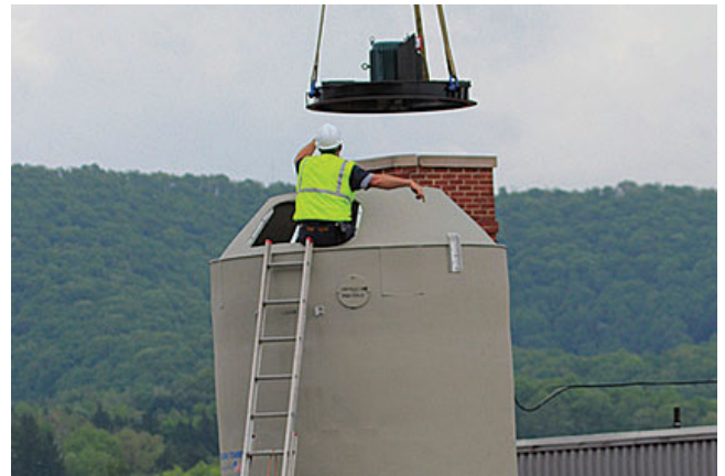
Davis Memorial Hospital in Elkins, WV, chose these plastic cooling towers in an effort to not only solve performance problems but also to protect against corrosion issues.
