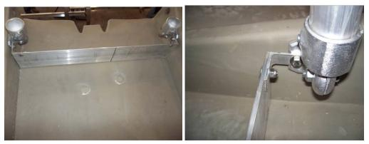
The kick-plate will be away from the ladder. Handrail fittings are already installed in place on the cooling tower. The handrail fitting has a set screw for securing the aluminum pipe.
