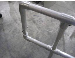
Match drill the ladder to the handrail.
