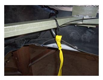
• Before installing PVC louver panels, verify that all post are correctly seated into the pockets of the tower body. Allow the upper housing to settle on the sump for at least 24 hours prior to installing the louvers.
