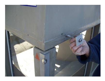
• Remove the temporary plastic "zip-tie" fasteners securing the above upper louver rubber deflector to allow the deflector to hang down. **DO THIS ONLY AFTER INSTALLATION IS COMPLETE.**
